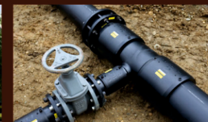
Under Ground HDPL Water Pipeline
